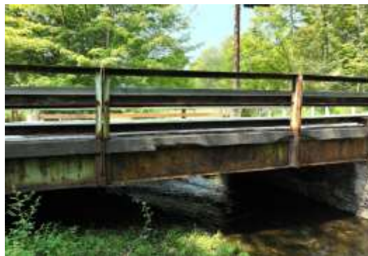
Figure 2: Hornbecks Creek bridge
