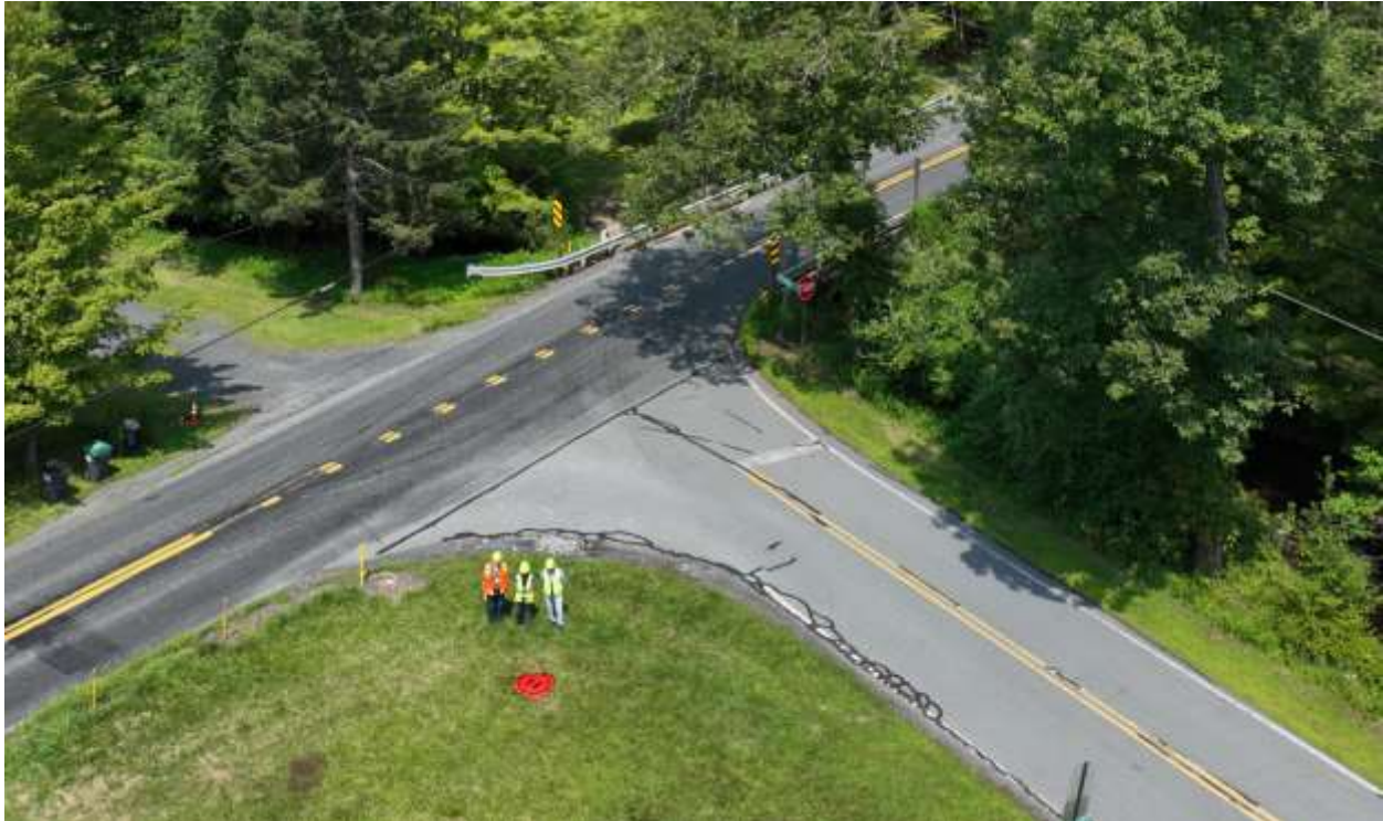
Figure 15: Intersection of SR 2001 with Chestnut Ridge Road (T-323) by Hornbecks Creek/Bridge
