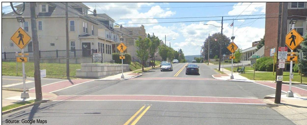
RRFBs are placed on both ends of a crosswalk and is a treatment option at many types of established pedestrian crossings. Research has shown a sharp increase in motorist yielding rates at marked crosswalks using RRFBs.
