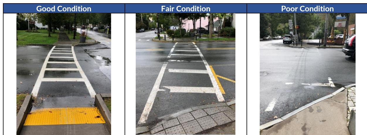
Overall, 22 crosswalks were found to be of good condition, 23 were found to be of fair condition, and six crosswalks were found to be of poor condition. The crosswalks with the most wearing and deteriorated conditions were located on the major roads (Broad Street and Harford Street) due to the high number of vehicles wearing down the crosswalk paint.
